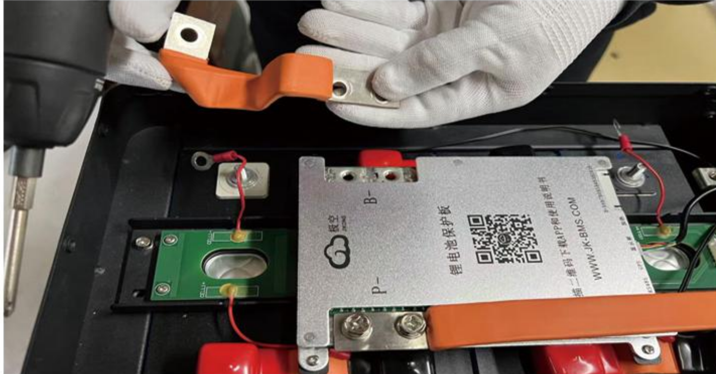
23. Place another special flexible busbar as shown in the figure.
