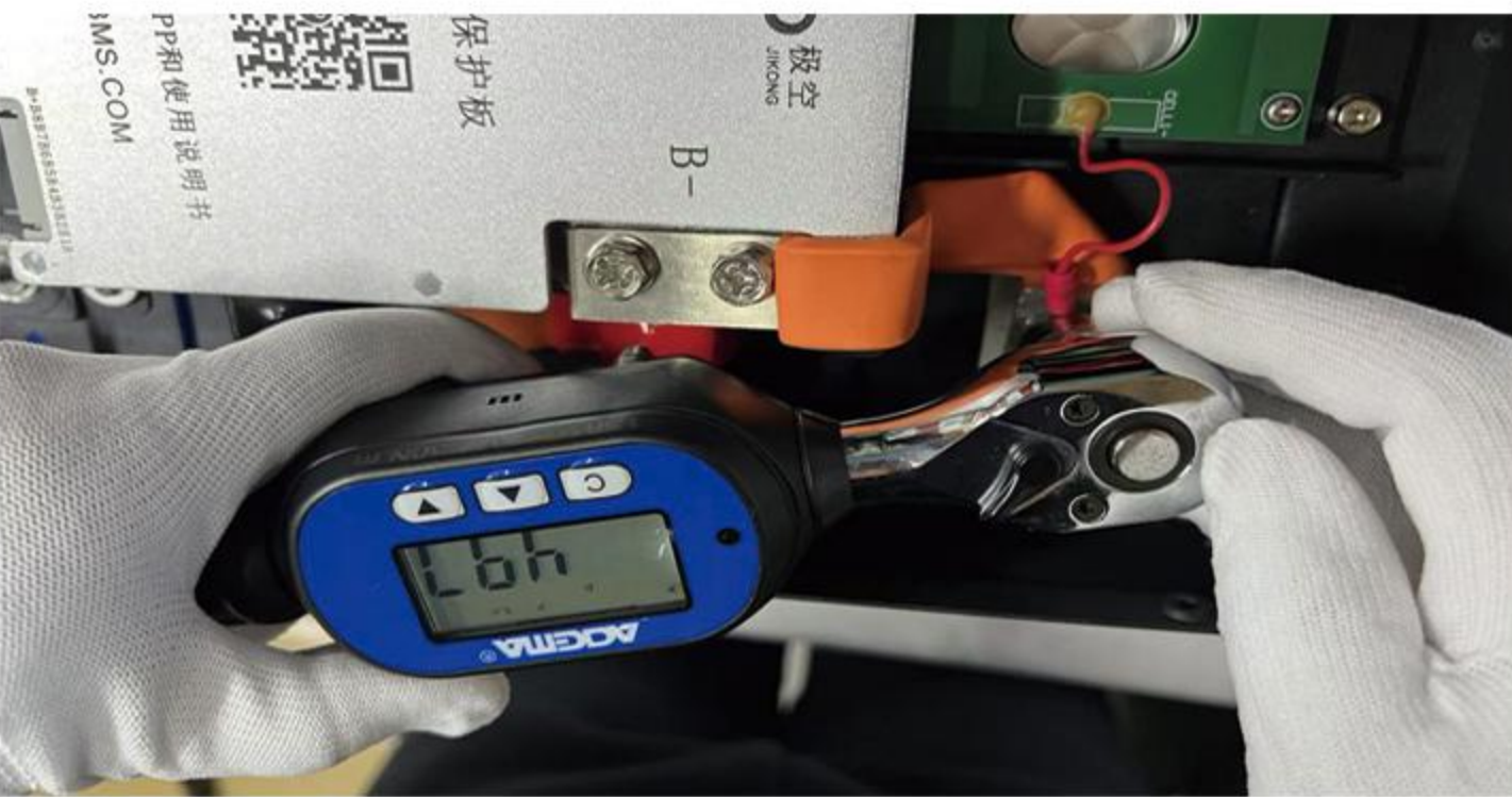
25. Tighten the screws at both ends of the busbar using a torque of 5 Nm.
