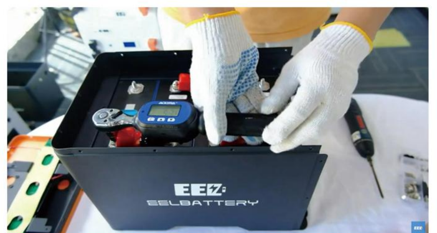
10. Tighten the M6 nuts with a torque of 5 Nm.
